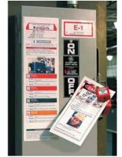
**Lockout:** A physical lock that holds a switch in the off position or holds shut a valve so hazardous energy cannot be released while the maintenance is occurring.
